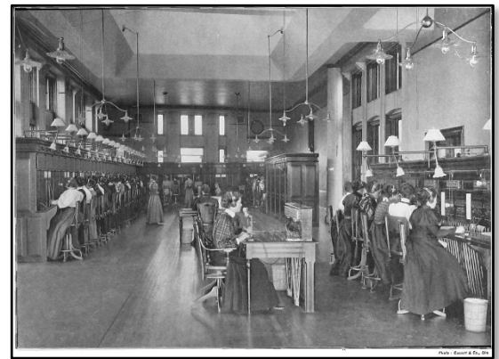
1888 Telephone Exchange, Montreal Canada
